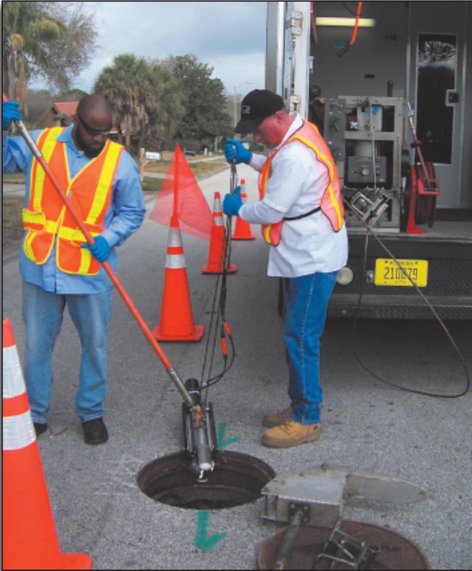
Tony Miles and Randall Britt lower the TV truck camera into a manhole to inspect the sewer main in a neighborhood as part of the proactive line inspection component of the city of Clearwater's CMOM program.
